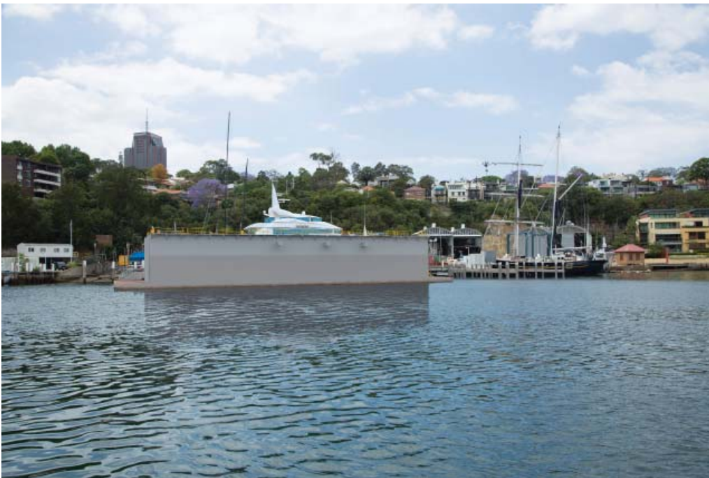
Position 4 (Map 2), Photomontage, FDD in closed condition, with vessel inside and acoustic curtains closed
