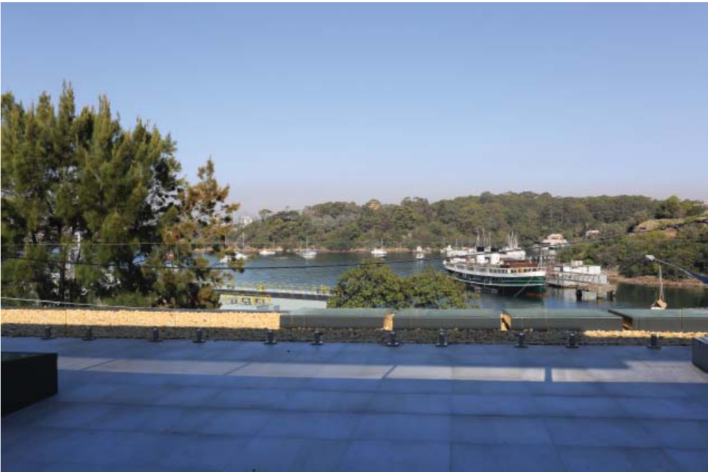
1_13 John St Terrace West side standing FDD in open condition with no vessel inside
