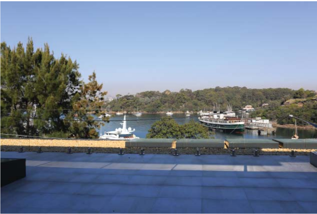
1_13 John St Terrace West side standing FDD in down condition with vessel inside
