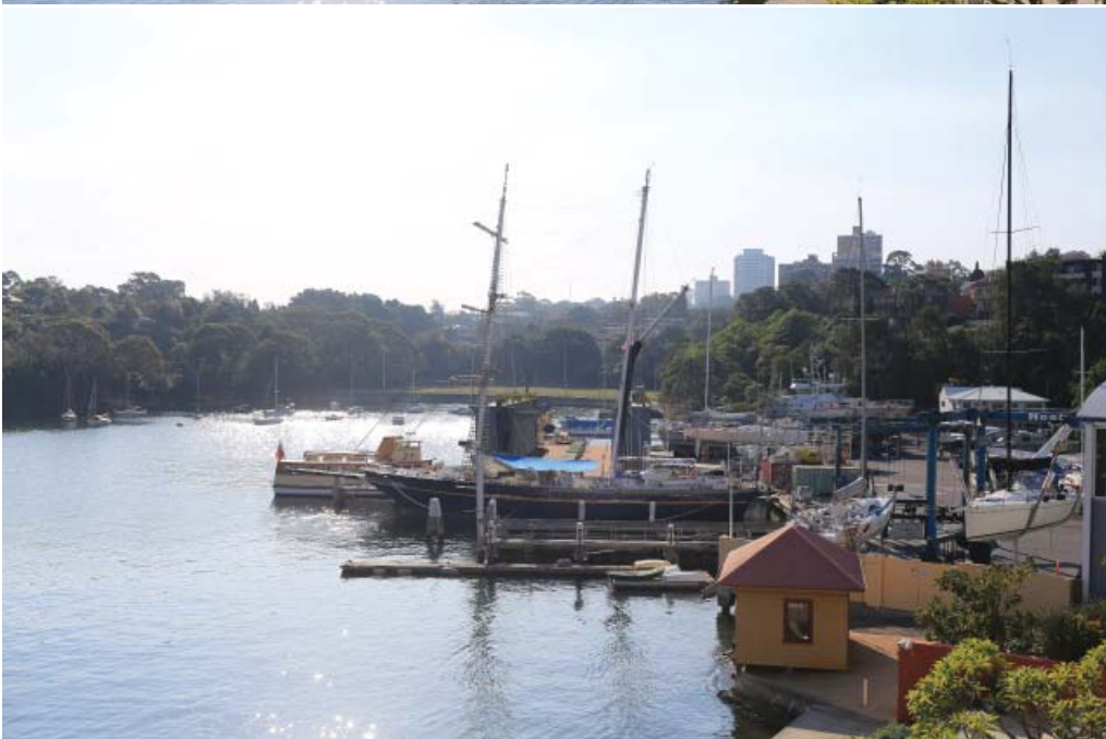
5_17 Munro St Lower floor balcony standing FDD in open condition with no vessel inside
