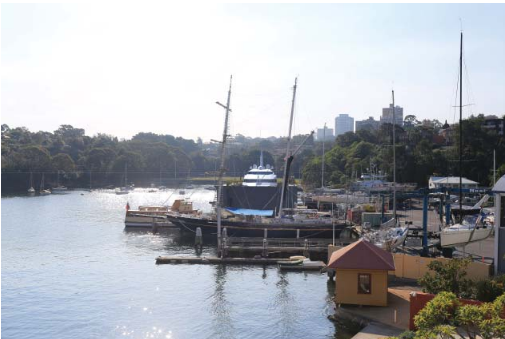
5_17 Munro St Lower floor balcony standing FDD in closed condition with vessel inside and acoustic curtains closed
